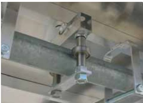
Tilt protection and guideway support
